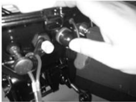
Internal fuel tank
